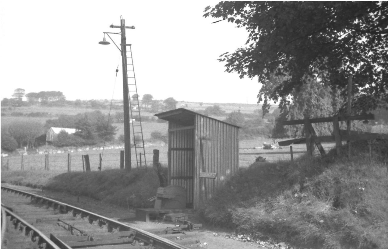
Callington Ground Frame that operated points 1a on the diagram
