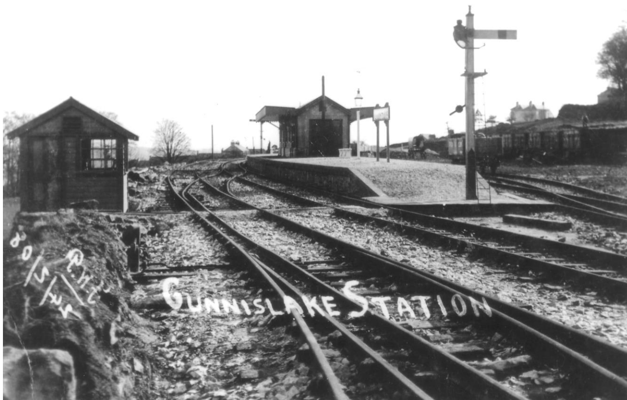
Gunnislake Station from the Callington end, May 1908. This photograph shows that not only does the location of the signal box differ from that in the drawings but the track layout has also been modified. The PD&SWJR signal at the platform end is mounted on a square timber post with a slight taper. Many of these were replaced in later years by Southern rail type signal posts.
