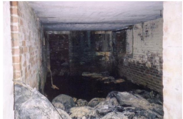
The interior of the Command post
