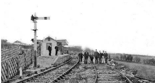
Gunnislake station track laying in 1907, note the Midland Railway style of fencing used by the PD&SWJR also visible below. The station buildings were designed by Holman Fred Stephens, later Colonel.
