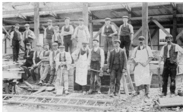
Callington Road Station under construction
