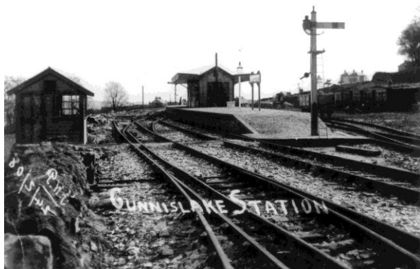
Gunnislake station May 1908 with the typical Stephens station buildings but still retaining the third narrow gauge rail in the siding
