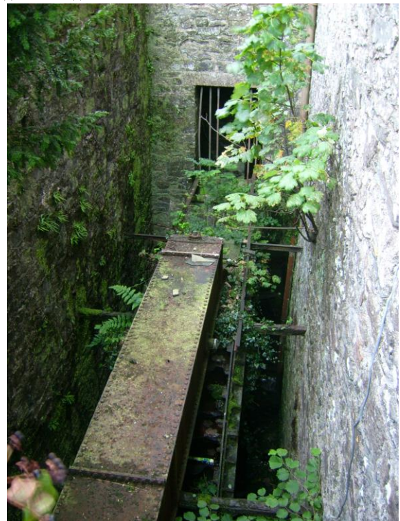
Water wheel pit
