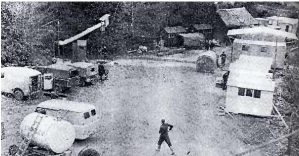
Work begins at Excelsior Tunnel c1960
