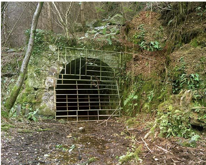
The tunnel entrance 1989. The entrance is now better secured.
