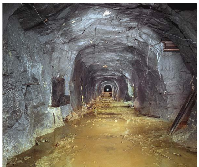
Looking along the full length of Excelsior Tunnel
