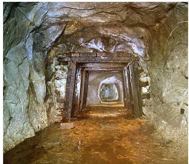
Timber props were used where the ground was unstable
